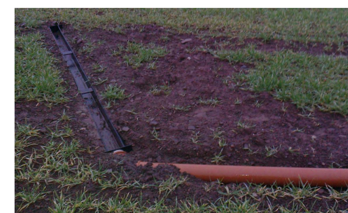
Gerlach trough installed across tramline
