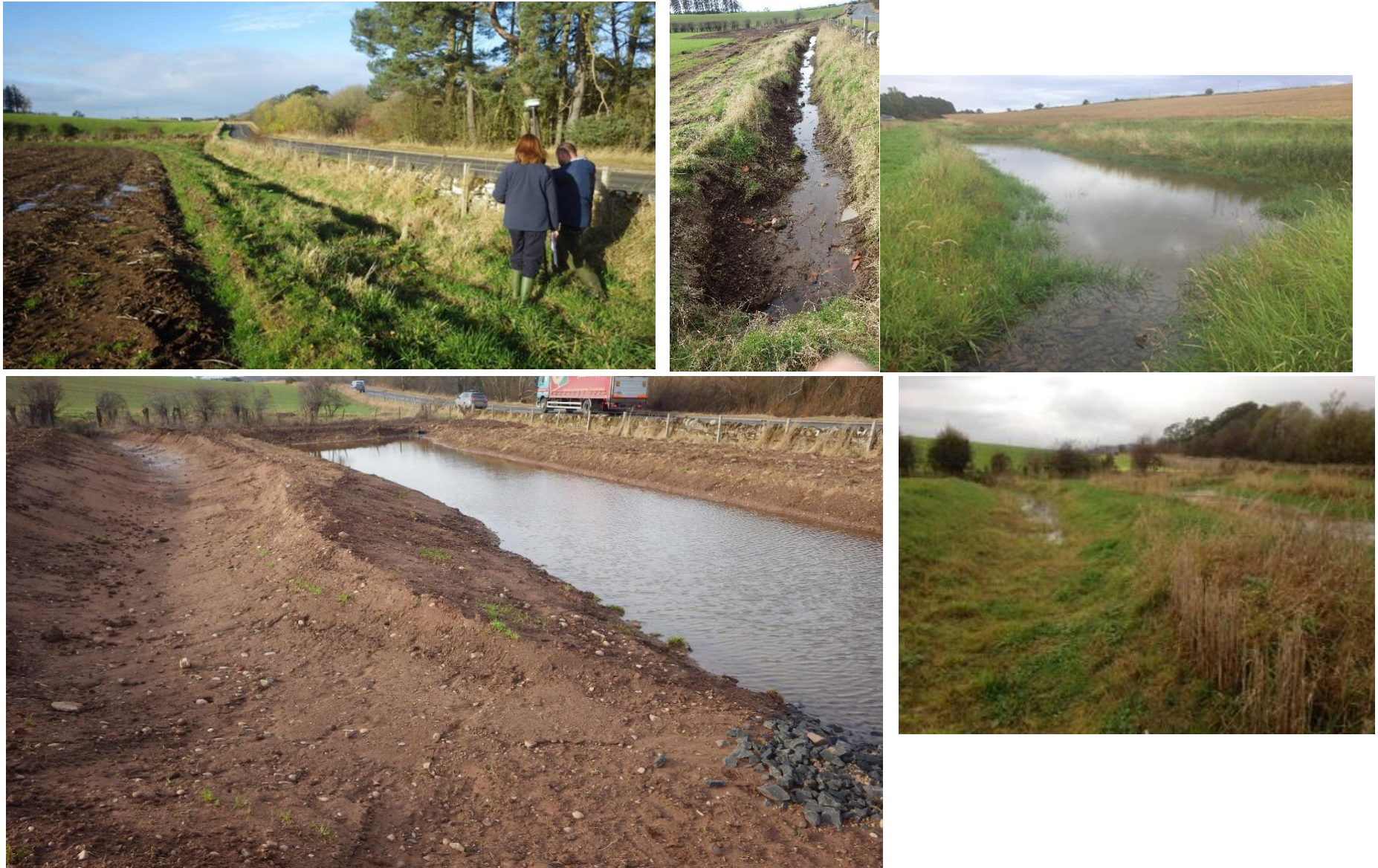
Figure 3. Site H in Figure 1. Swale and sediment trap/wetland installed at Greenhead Farm, upstream of Fonah Bog with AECS funding (2018). (a) prior to installation (b) ditch capturing burst drain (c) swale inlet from ditch (at back of picture) and sediment trap (water filled after storm event) with outlet to culvert under road. (d) summer 2019 view of wetland (e) Nov 2019 view of swale.
