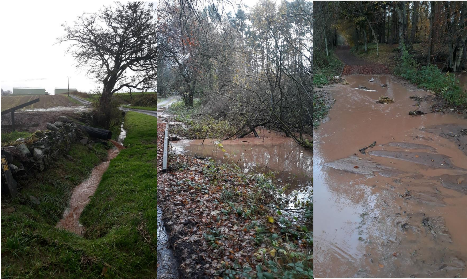
Fig 6. Impacts of runoff this autumn from bund where work is in progress on SWT site (Fonah Bog)
