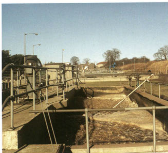
Waste Water Treatment Plant
