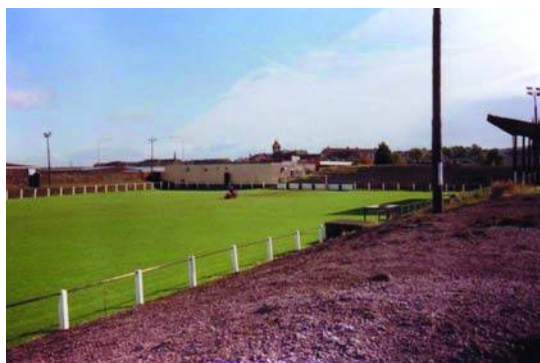
Plate 2b Terracing around the football pitch has been built from chromite ore processing residue
