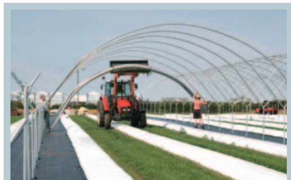
Construction of Spanish tunnels
