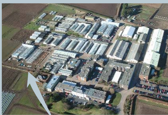
Aerial view of new general-purpose glasshouse complex.
