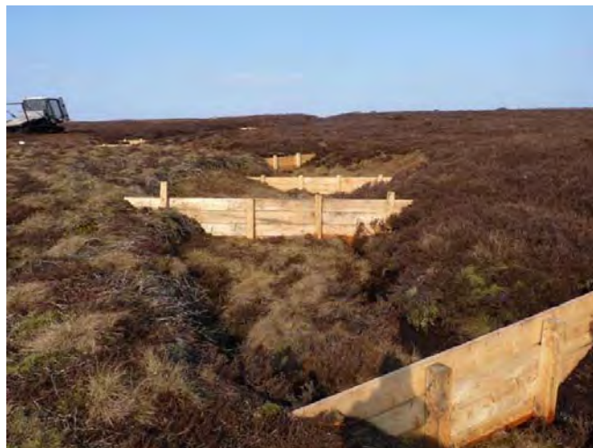
Blocking ditches, channels, gullies
