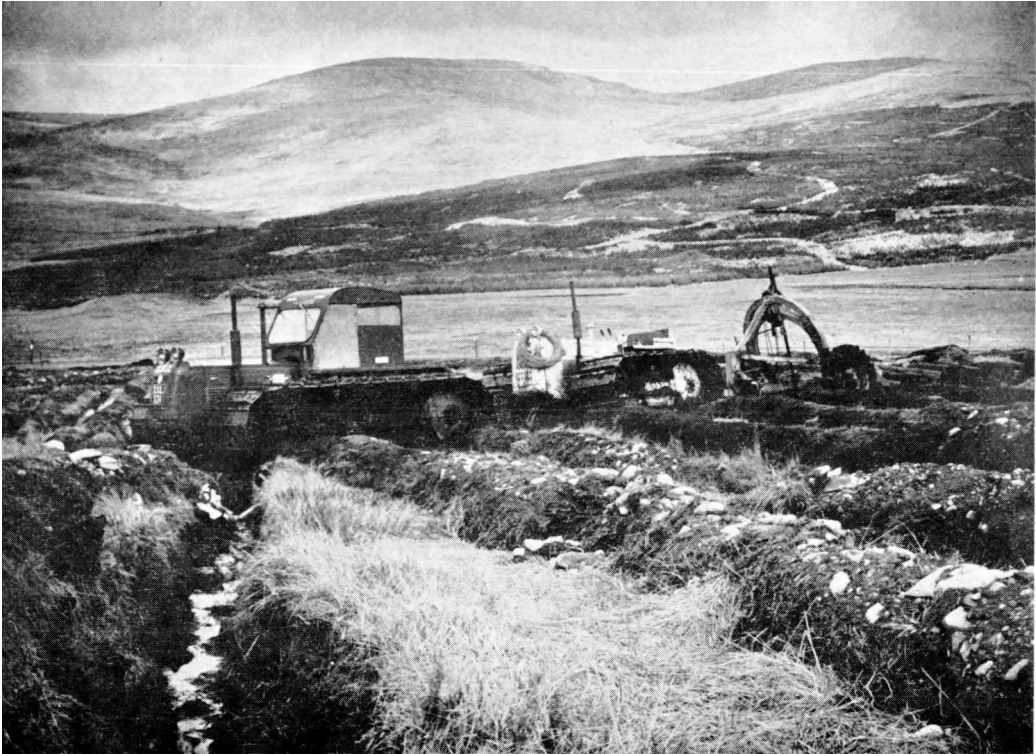
PLATE 11/Crawler tractors being used in tandem for the intensive drainage of shallow peat prior to afforestation. Shalloch on Minnoch Hill in the background rises to 2520 feet.
