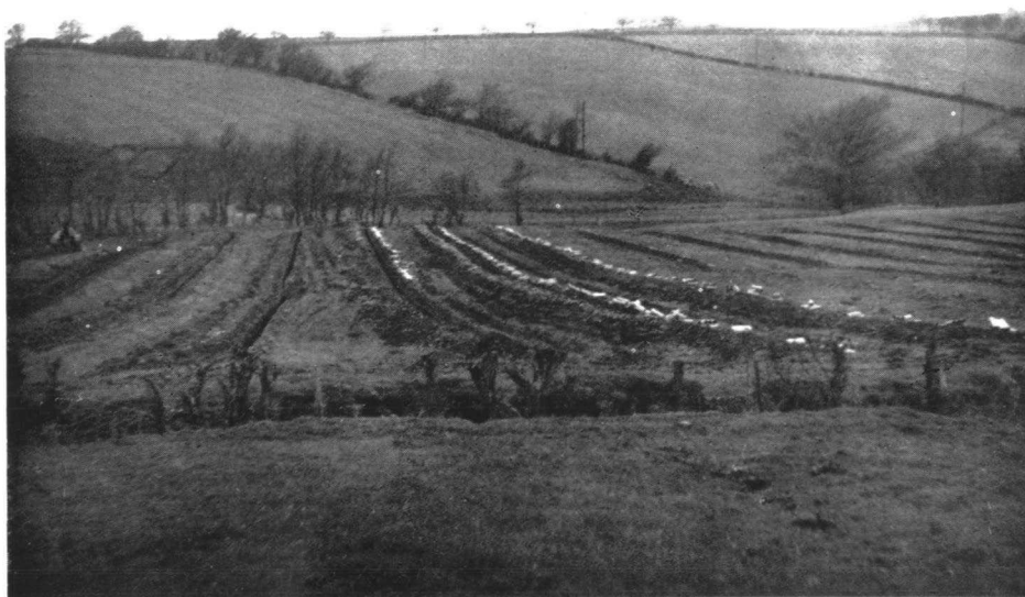
PLATE 8 Tile-draining on poorly drained site in Lowland Transition Zone near Sorn. Sorn association. Note rigging and furrowing in the background.
