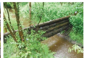
6) Leaky dams/barriers are being installed across streams
